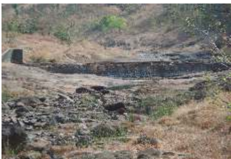
Construction of a check dam
